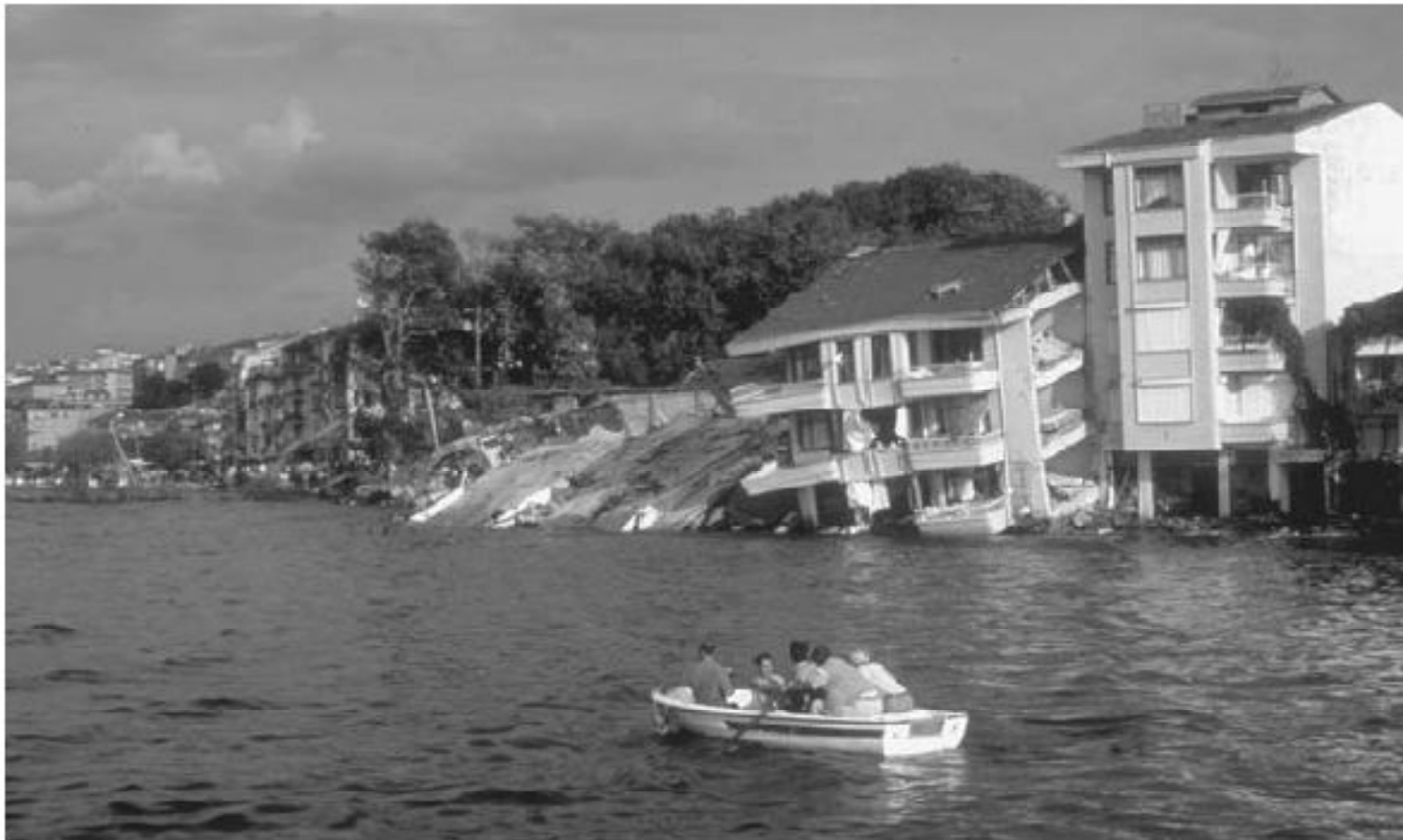
FIGURE 7.13 Subsidence and lateral spreading due to liquefaction lead to the collapse of buildings along the shoreline in the fishing village of Guzelyali during the 1999 Turkey (Kocaeli) earthquake. (J.C. Borrero photo, courtesy National Oceanic and Atmospheric Administration-National Geophysical Data Center)
