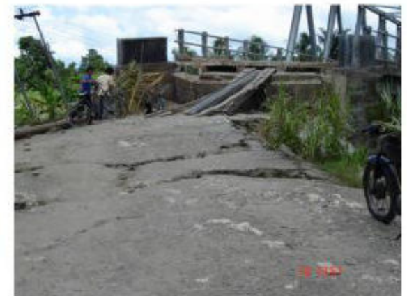
Fig.8.3 Liquefaction induced damage to Muzoi River bridge by 2005 Nias earthquake
