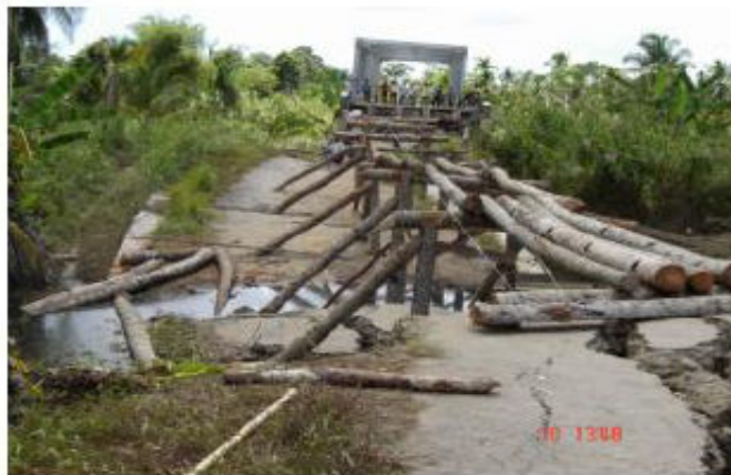
Fig.8.3 Liquefaction induced damage to Muzoi River bridge by 2005 Nias earthquake
