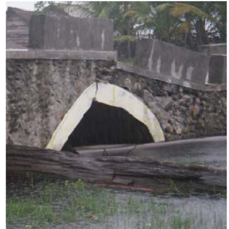
Fig.5.9 Damage to the arch bridge at Pasir Gantung due to ground liquefaction
