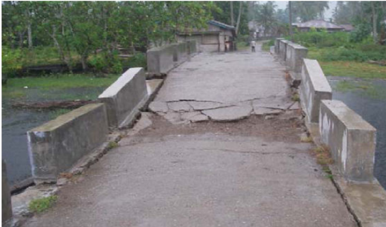
Fig.5.9 Damage to the arch bridge at Pasir Gantung due to ground liquefaction
