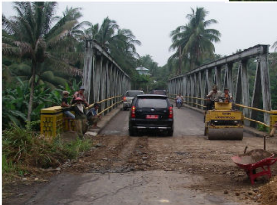
Fig.5.11 Damage to approach embankments of bridges
