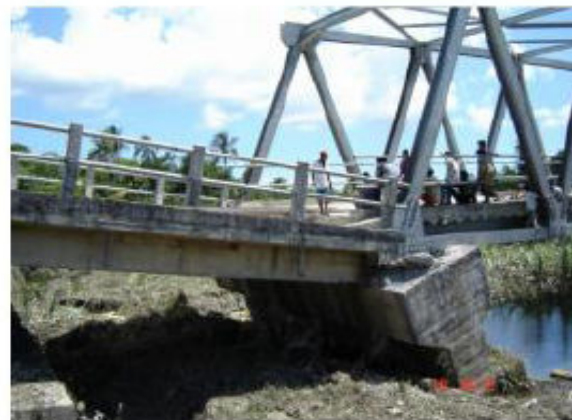
Fig.8.3 Liquefaction induced damage to Muzoi River bridge by 2005 Nias earthquake
