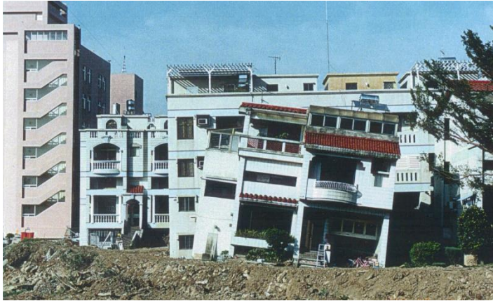
Liquefaction and settlement
