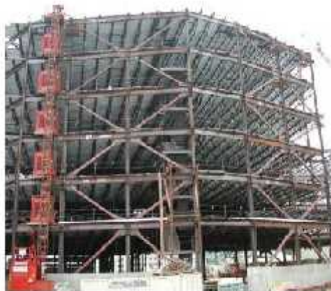
Figure 2.1 Bracing at The Building Structure
